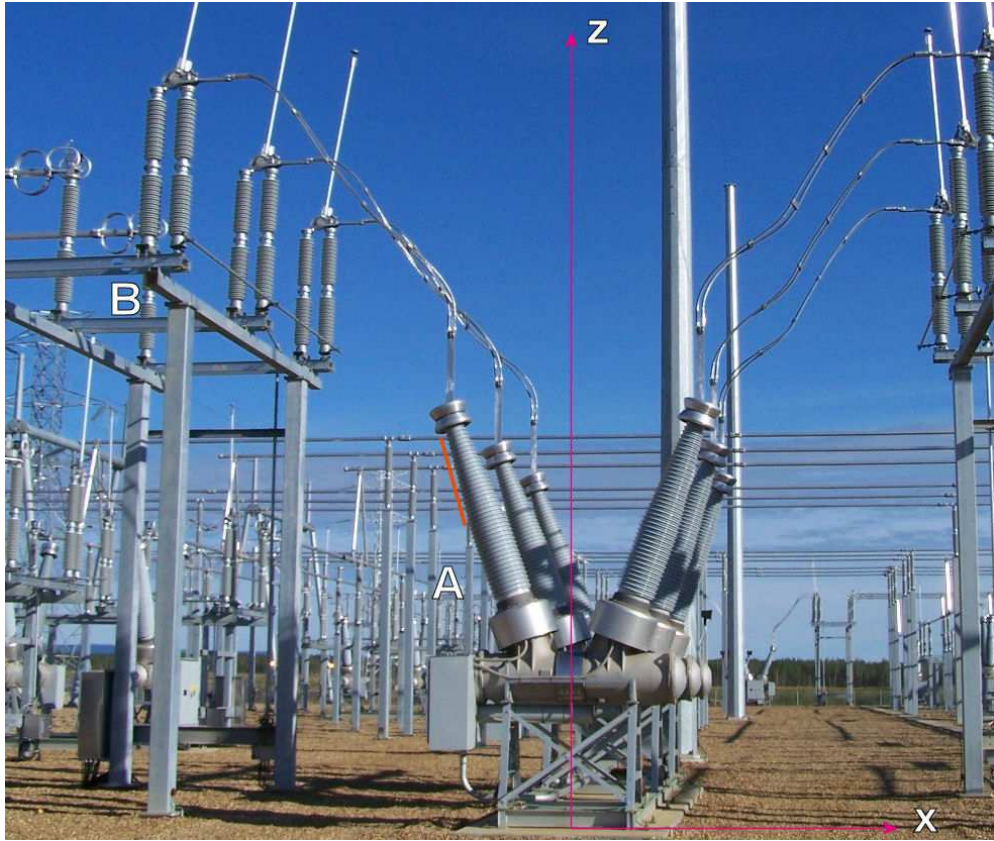
Figure 1: Circuit-breaker system with model coordinate system. A ) Busing (height 2.7 m). B ) Grounded base of the disconnect switch. Orange line shows the path for electric field scans.
